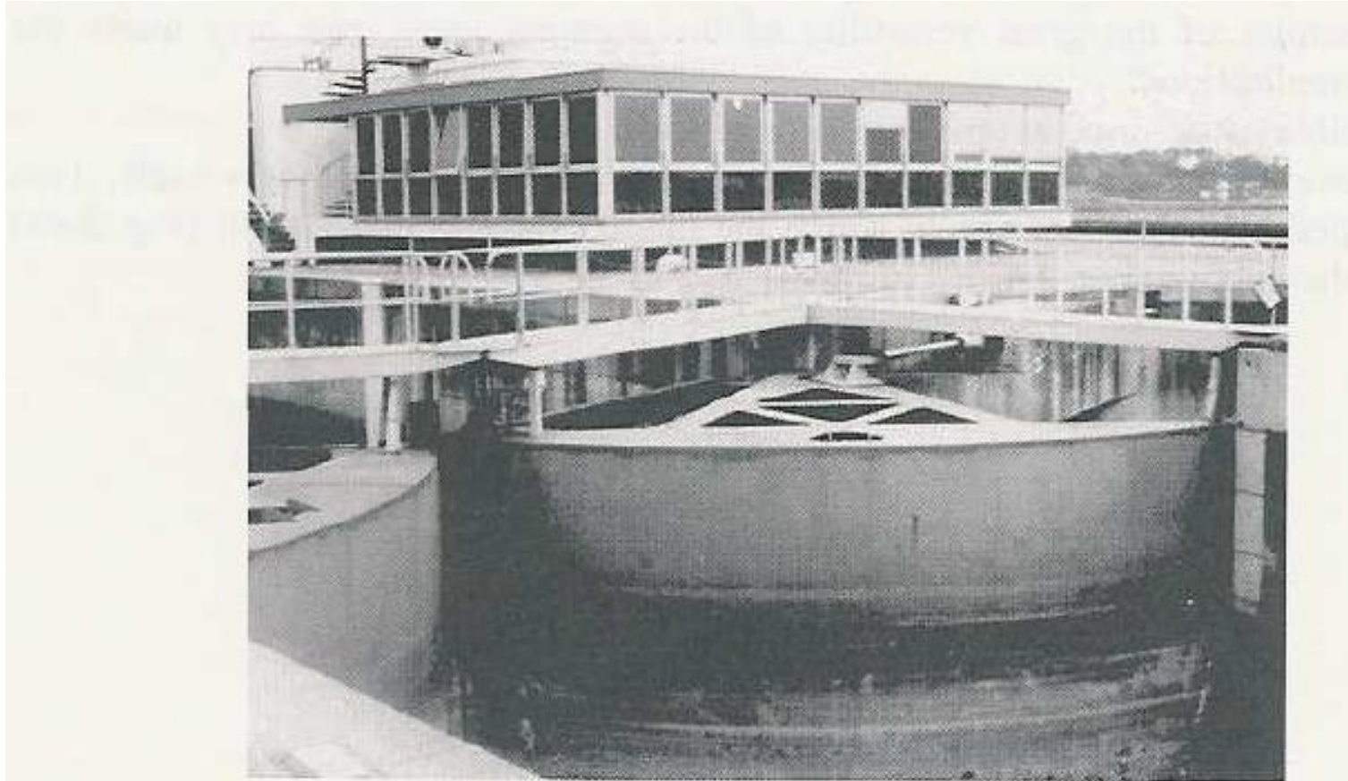
Fig. 2.46 Segment gate with vertical axis of rotation, Saint-Malo lock
