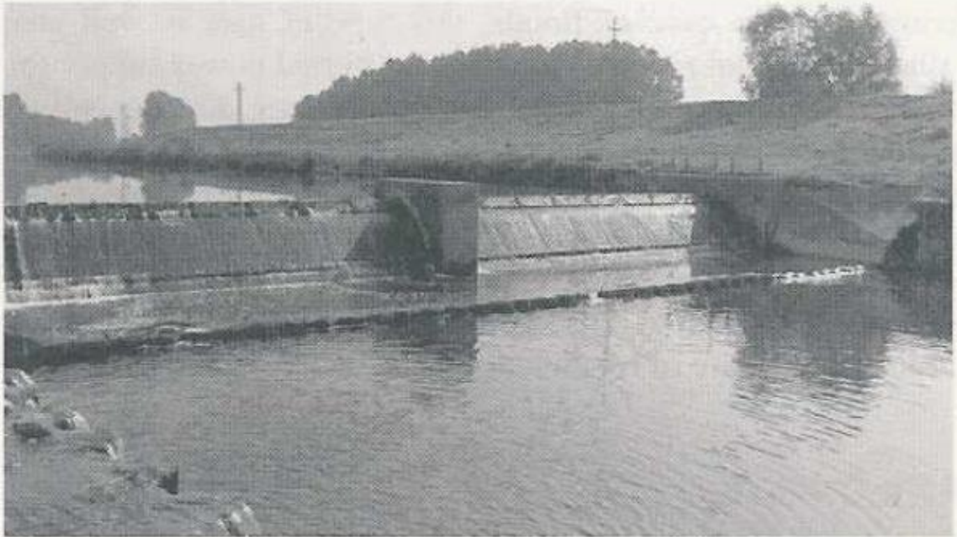
Fig. 2.75 Bear-trap gate, Fröndenberg Power Plant, 15.5 m wide by 1.5 m high
