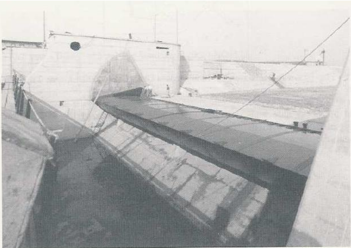
Fig. 2.7 Flap gate, Ottendorf Dam (M.A.N.), 30 m wide by 5.5 m high
