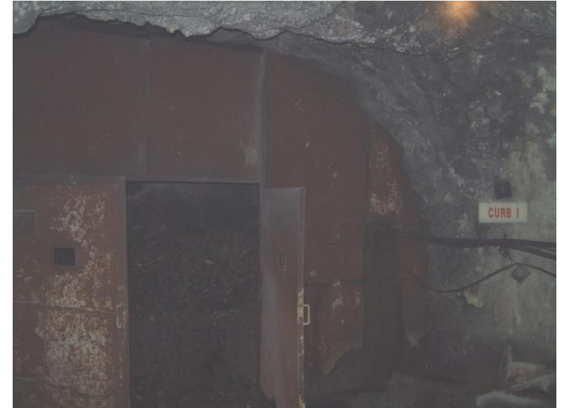
(iii) CURB-1 ( \pm 54,3 \text{ m}^3/\text{s} ); diameter 2,5 m
